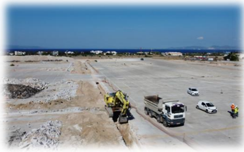
Figure 1: In situ chemical oxidation; Bioremediation on site; removal of hazardous and non-hazardous waste (pipelines, tanks etc)
